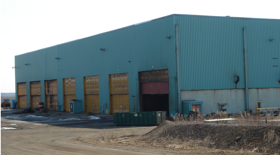
Figure 20-5 Area 1 Truck Shop from the north west showing the six haul truck maintenance bays and truck wash down bay (nearest camera).
